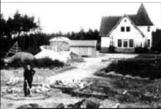
Frič on foundations of the central cupola, year 1908.
